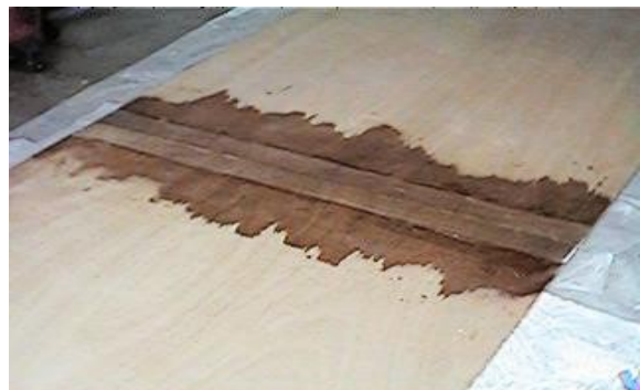
Fig.6. Jointing with the help of glass cloth
